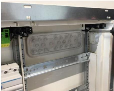
Dust-tight flange VZ741 mounted on the rear of the enclosure
